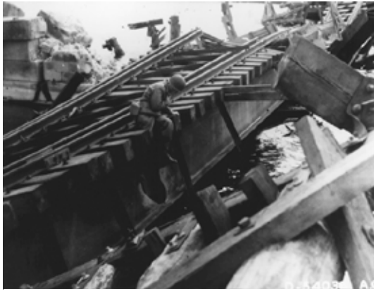
A GI gazes into the water from a railroad bridge destroyed by tactical bombing. Courtesy National Air & Space Museum, Smithsonian Institution
